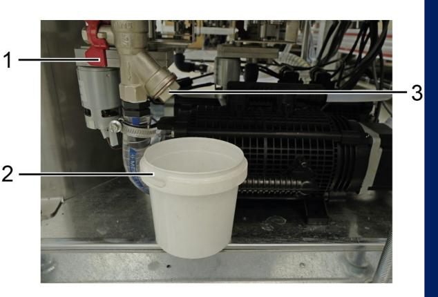
Close the key before the filter (1); Place a container under the terminal part of the filter (2); Unscrew the cap containing the filter using a 22 mm wrench (3); Remove the filter and clean it with running water; Reassemble the filter and the corresponding screw cap, then open the circuit by inserting the key;
